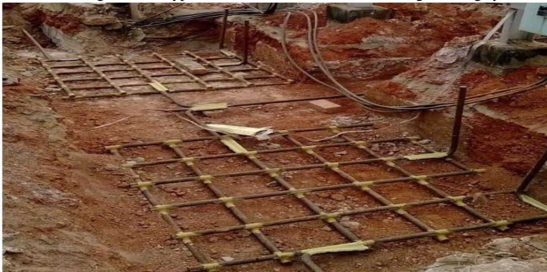
Figure 1. Typical Substation Earth Mat [Study Electrical, 2014]
